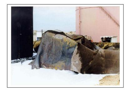
Fig. 2 – The Roof in the Dike
