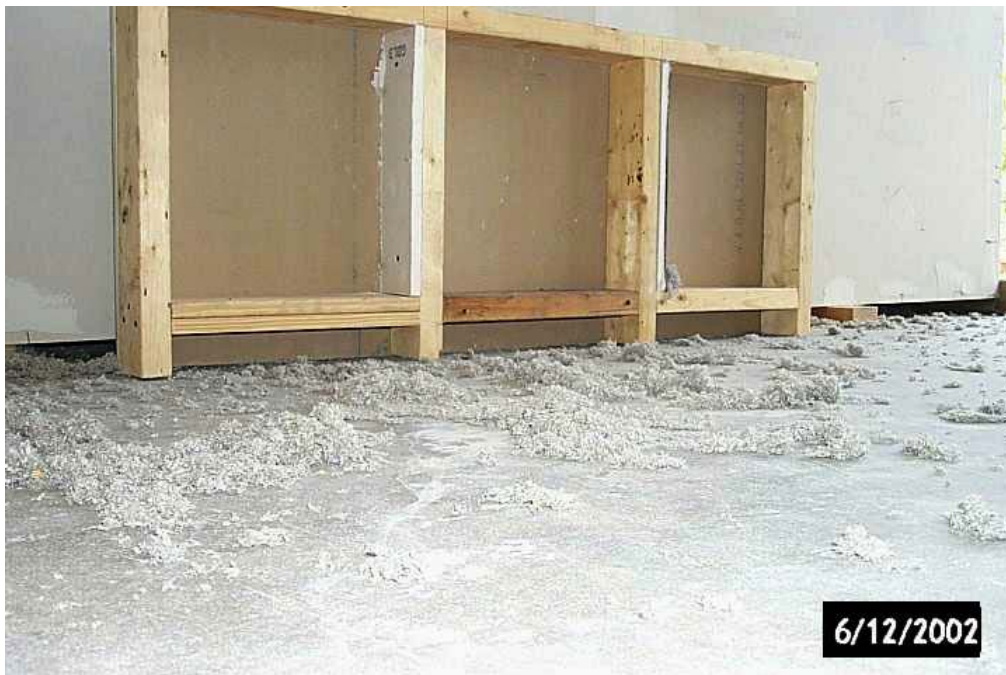
One of the wall sections prior to insulating the center cavity
