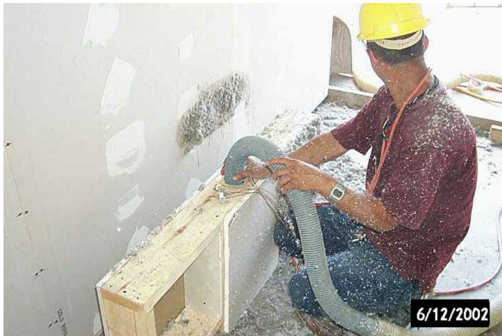
One cavity was dry-filled through a hole in the top plate
